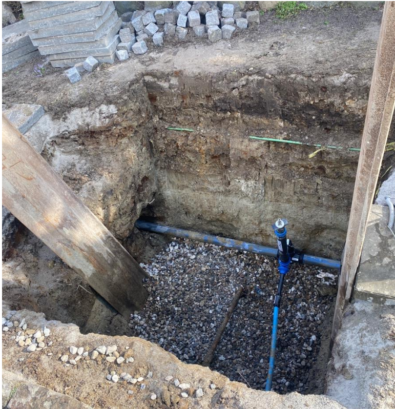
Figure 2 - Trench with new valve system
